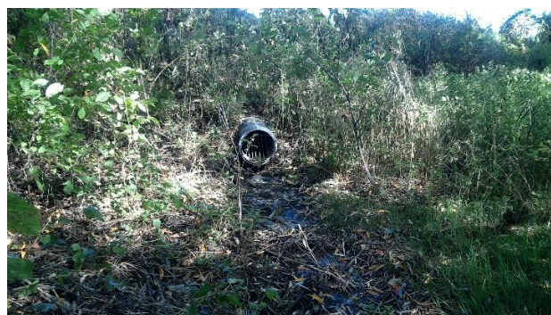
Photo 10. Outlet of tile drain for Tributary E at County Road 47 (September 25, 2019).
